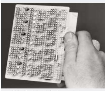
SMS, or Standardized Modular System, technology replaced vacuum tubes.
