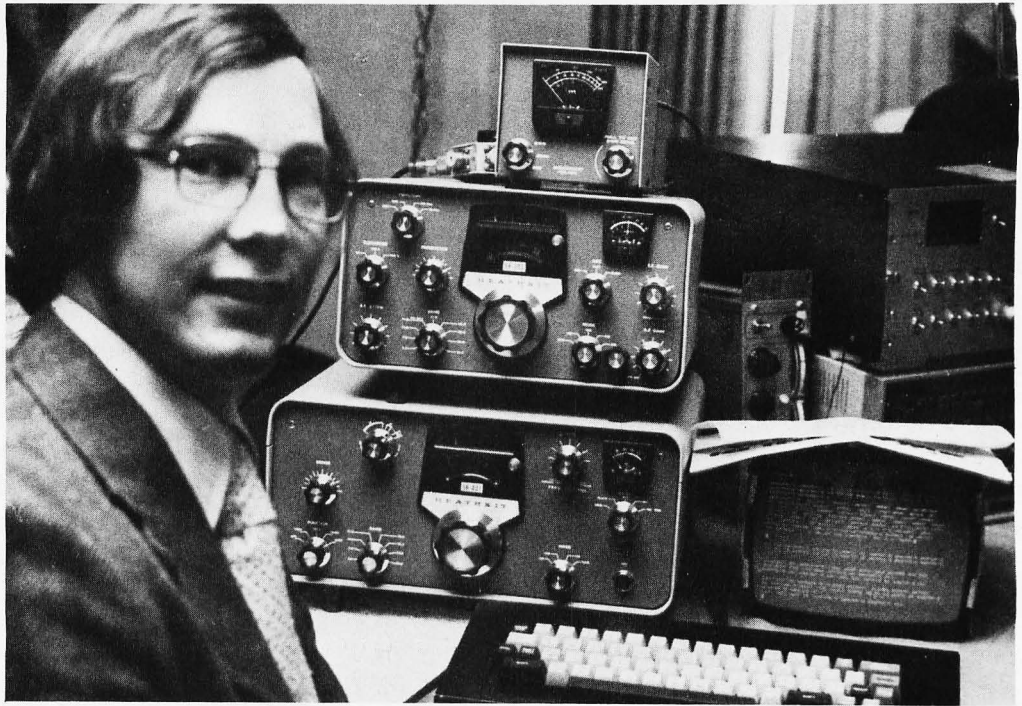
Don Alexander of Columbus OH was named the grand prize winner in the MITS World Altair Computer Convention demonstration contest. Don is shown here with his computer controlled amateur radio Teletype station. The radio equipment is the stack at the left. At the right is his homebrew video display output on an OEM monitor, and in the background at the right is his Altair 8800 on top of which is perched the radioteletype converter unit. The station is completed by the keyboard unit in the front, and a Model 19 Teletype machine (only a corner is visible at right) which logs station contacts during contests.
